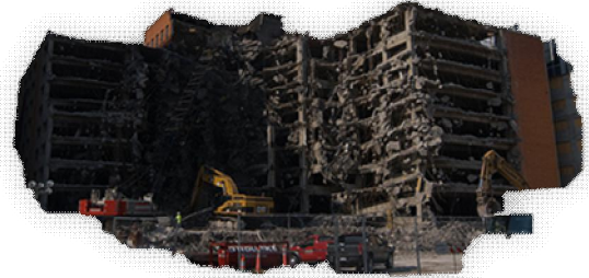
Fig. 2. Demolition of 7 to 9-story Parking Garage
